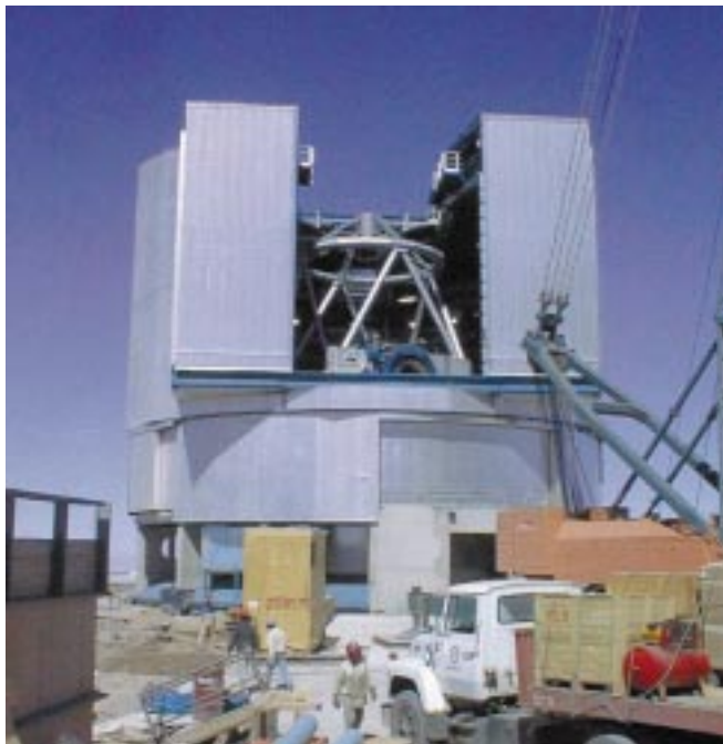
Figure 1: A recent view of Unit Telescope 1 through the open slit doors in the upper rotating part of the enclosure. ◀
