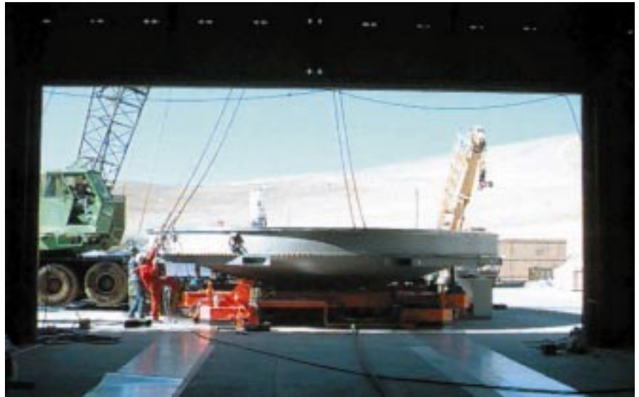
Figure 3: View from the inside of the Mirror Maintenance Building through the 10-m door. The lower part of the coating plant has been placed on the air cushion transport system which will move it along the two tracks seen in the foreground. The total moving weight with an 8.2-m mirror in the chamber is about 50 tons.
