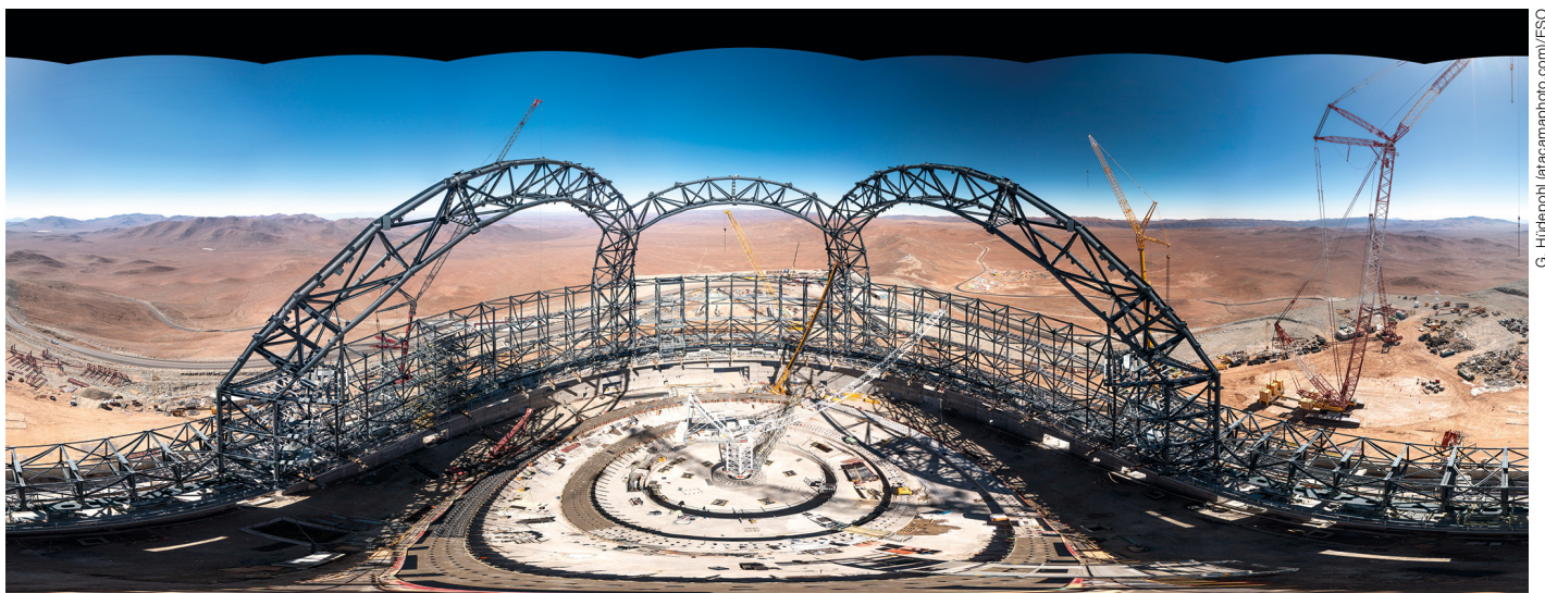
A panoramic view taken from the top of the dome of ESO's Extremely Large Telescope (ELT) in early August, 2023. When completed, the dome will be 80 metres high, weigh more than 6100 tonnes and rotate 360 degrees on 36 trolleys.
