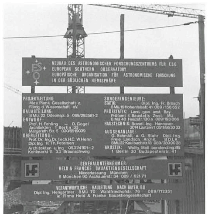
At the entrance to the construction site. ►
