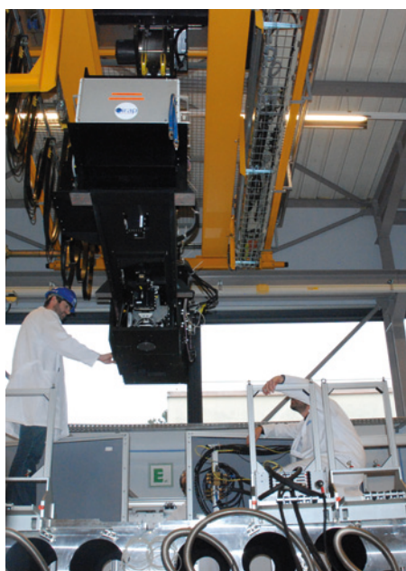
Figure 6. The fore-optics system attached to the integration hall crane can be seen before its descent onto the main structure.
