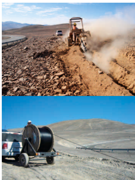
Figure 2. Two views of the work involved in laying the EVALSO optical cable from Paranal to link with the existing network infrastructure; upper image: cutting the trench; lower: laying the cable in the trench.
