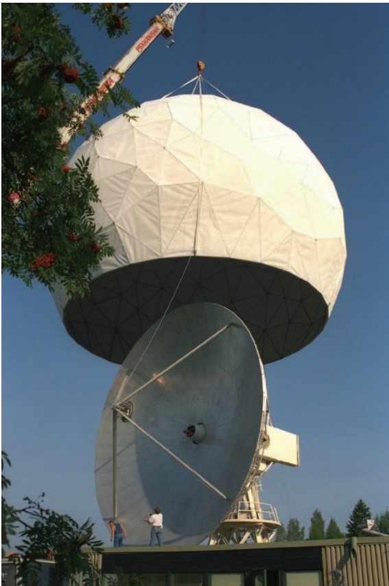
Figure 2: The 13.7-metre radio telescope of the Metsähovi Radio Observatory, Helsinki University of Technology, is enclosed within a 20-metre radome that protects the telescope from rain, snow and wind. The surface accuracy of the telescope is 0.1 mm (rms). The observing frequencies available at Metsähovi range from 2 to 150 GHz, the lower end being used for geodetic VLBI and the higher end for millimetre VLBI. The primary observing frequencies, however, are in the mid-range, 22 and 37 GHz.
