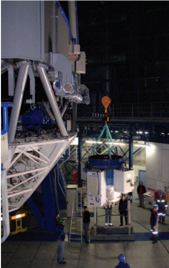
Figure 4: SINFONI during installation at UT4. The SPIFFI cryostat vessel is the grey aluminum part below the AO-Module (blue). To the left, the M1 cell of the VLT.
