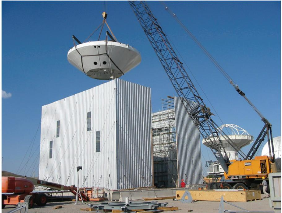
*The mounting of the BUS onto the antenna at the ATF site.*
