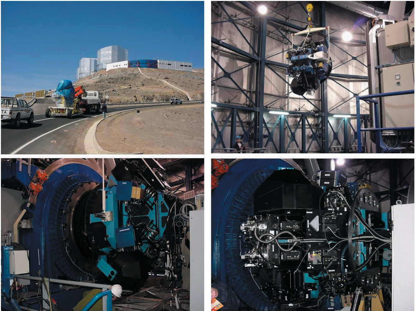
Figure 2: Installation of VIMOS on the VLT-UT3. From upper left, clockwise: (a) transportation of VIMOS from the Paranal Observatory integration facility to the telescope, (b) VIMOS being hoisted inside the dome of Melipal to reach the Nasmyth platform, (c) installation on the Nasmyth rotator, (d) VIMOS after cabling and co-rotator installation.
