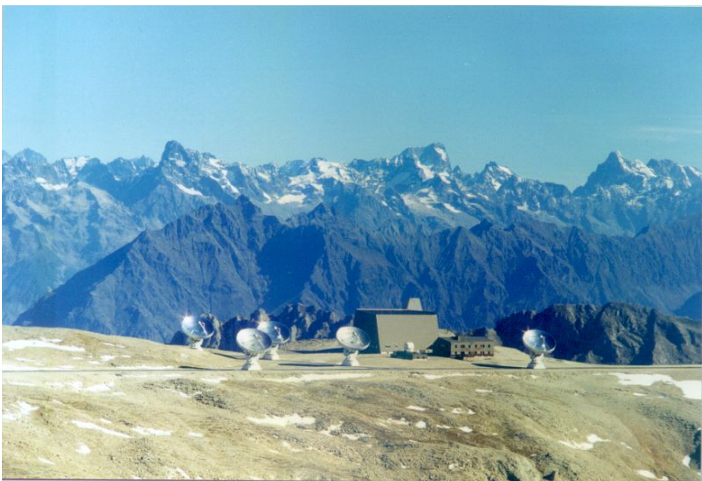
IRAM array (oct. 1999, courtesy S.Muller). Plateau de Bure (french Alps, 2550m). Area = 880\text{m}^2 (5Ant.). Best Resol. = 0.5'' at \delta \simeq 30^\circ . Dual Frequency receivers 85-115 GHz (3mm) & 208-248 GHz (1.3mm).
