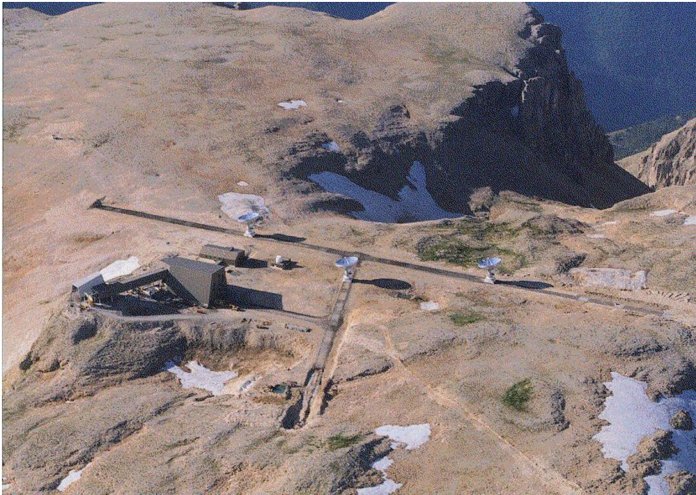
IRAM array (june 1997, copyright IRAM). The E-W track is doing an angle of \sim 15^\circ with the west. Baselines are: N-S = 232m, E-W=408m.
