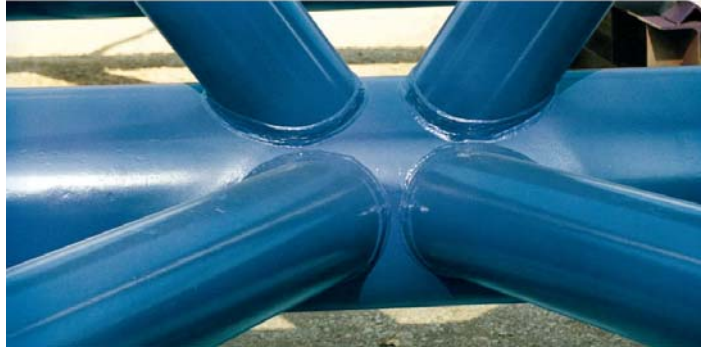
Figure 9-15: Typical welded node.
