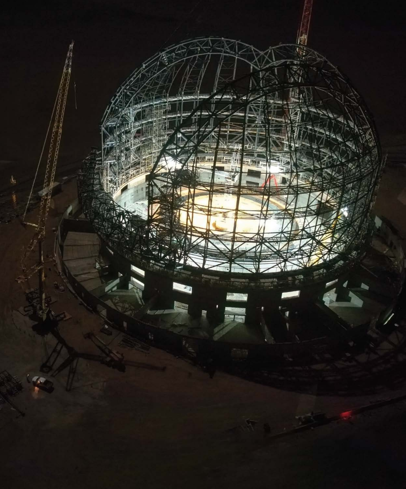
This drone image, taken in late September 2023, captures an aerial view of ESO's Extremely Large Telescope (ELT) dome at night-time. It already has the recognisable spherical shape of a telescope enclosure with the construction of the frame well on its way to being completed by the end of 2023.
