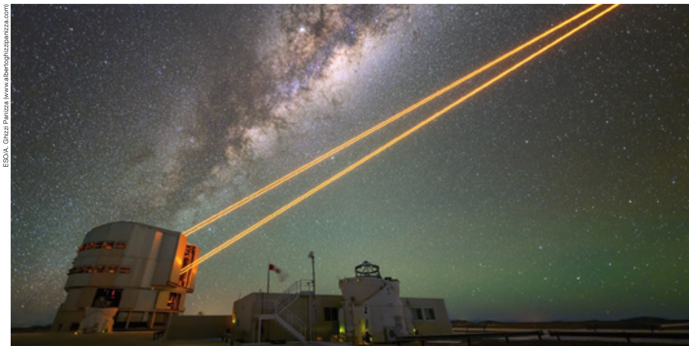
This image depicts the four powerful laser beams leaving Unit Telescope 4, or 'Yepun', at ESO's Very Large Telescope (VLT) in Chile's Atacama desert. These form the VLT's 4 Laser Guide Star Facility,
