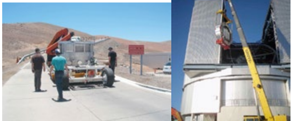
Figure 2. KMOS cryostat on the road from the integration hall to the summit (left); the CACOR being hoisted into the dome of UT1 (right).
