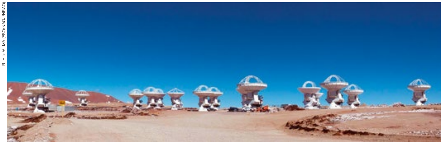
Figure 1. Seventeen ALMA antennas on the Chajnantor plateau, when fringes on 136 baselines (between the 17 antennas) were obtained for the first time. The first antenna to the high site produced by the AEM consortium was included in the array and is visible near the centre left of the picture.
