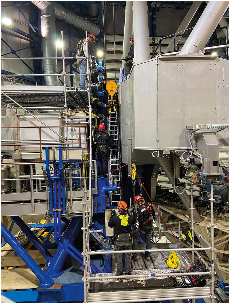
Figure 7. Implementing the upgraded cable wrap at Nasmyth B on UT2 in June 2023.
