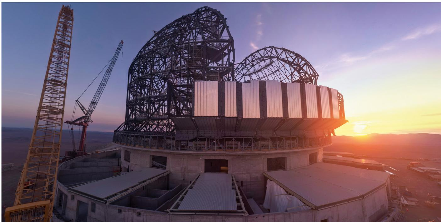
ESO's Extremely Large Telescope (ELT) is quickly coming together before our eyes. In this webcam image over Cerro Armazones in Chile from 16 February 2024, the setting Sun illuminates the first pieces of cladding installed on the ELT dome. The hemispheric structure
