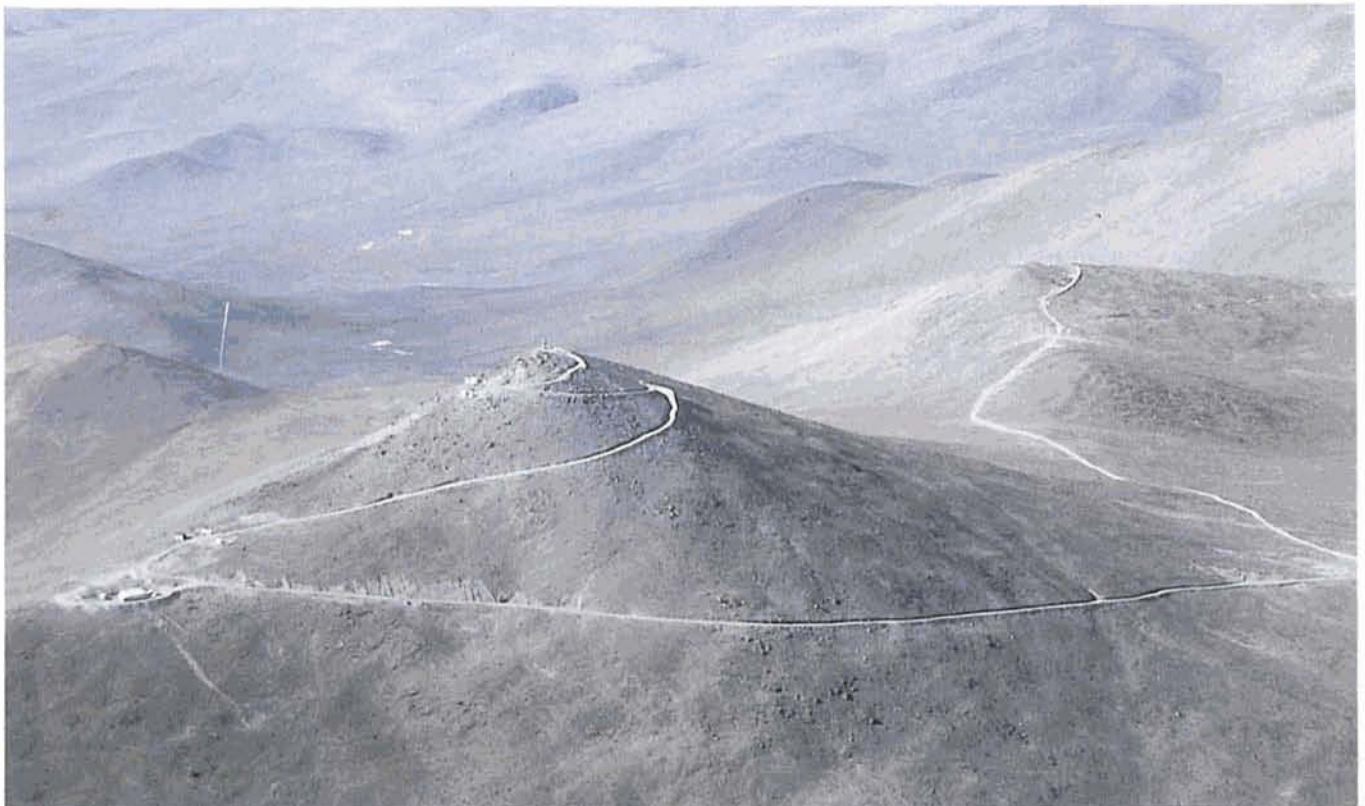
This aerial picture of Cerro Paranal was taken in late 1990 from the south. The Pacific coast is to the left, at a distance of 12 km. The constructions at the left are the living quarters for the site survey team, in place since 1983. On the top of the mountain various instruments are installed which permanently monitor the atmospheric quality and perform meteorological measurements.
