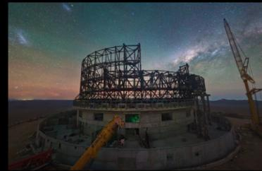
This image shows a webcam view of the construction site of ESO's Extremely Large Telescope at Cerro Armazones, in Chile's Atacama Desert. At the time the photograph was taken, in June 2023, engineers and construction workers were assembling the structure of the telescope dome.
