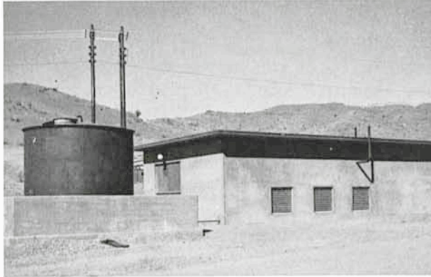
Fig. 2: Power Plant with its oil tank in Campamento Pelicano.
