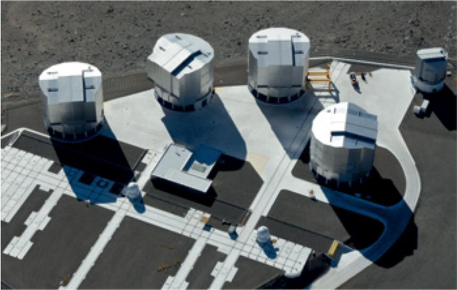
*By 1992, the VLT had assumed the shape that we know today, seen here in this aerial photo: The four 8.2-metre Unit Telescopes in their enclosures, placed in an almost trapezoidal configuration, with the movable 1.8-metre Auxiliary Telescopes on tracks, the interferometric focus building at the centre of the photo and the control room building to the left, below the telescope deck. A comparison with the illustration on p. 200 shows how much it had changed. (Photo: Gerd Hühdepohl)*
