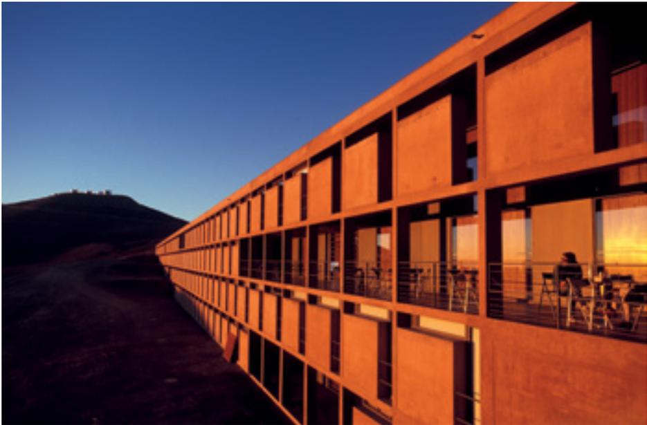
*The 167-metre-long façade of the Residencia faces the Pacific Ocean with its impressive sunsets that makes the ferrous oxide pigmented concrete walls glow. The building covers a total of 12 000 square metres. It was constructed by the Chilean company Vialy Vives at a total cost of 12 million euros. (Photo: Gerd Hüdelpohl)*
