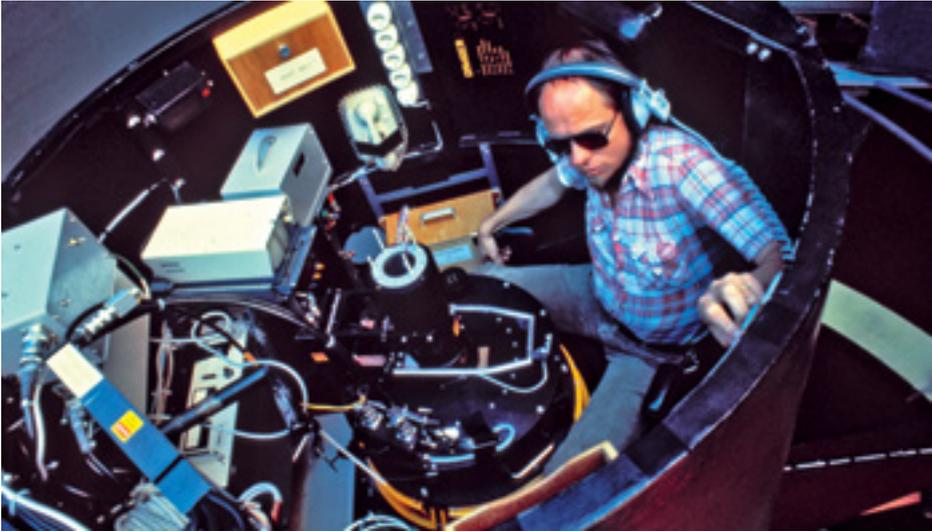
*Gerhard Schnur riding in the prime focus cage at the top of the 3.6-metre telescope. From this position, the observer guided the telescope and exchanged the photographic plates. (Photo: John Launois/Black-Star)*
