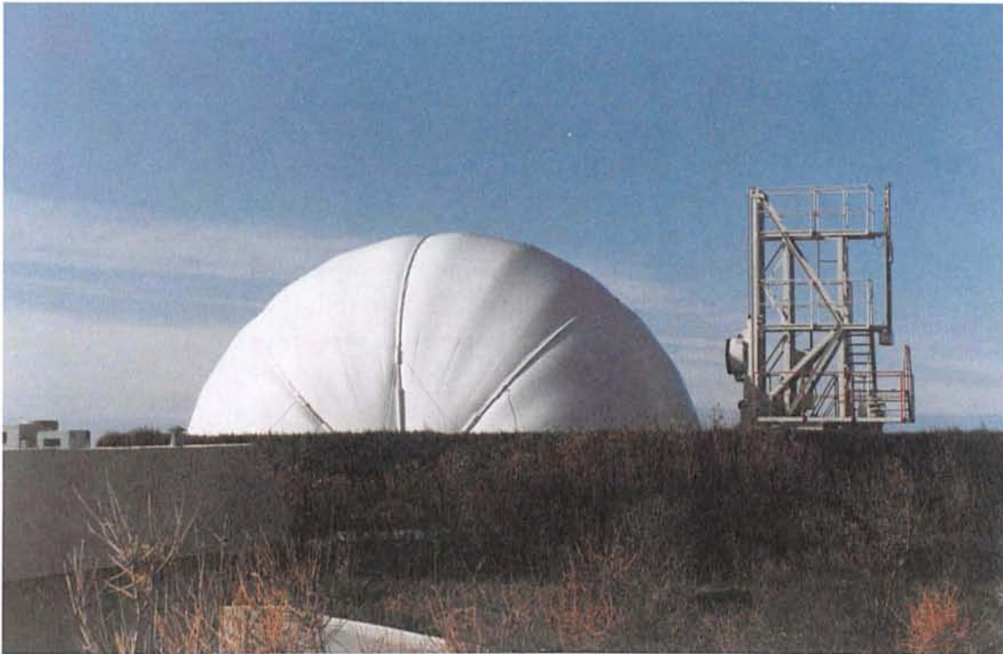
Figure 8.9: Photograph of an existing inflatable dome similar to the one proposed for the VLT.
