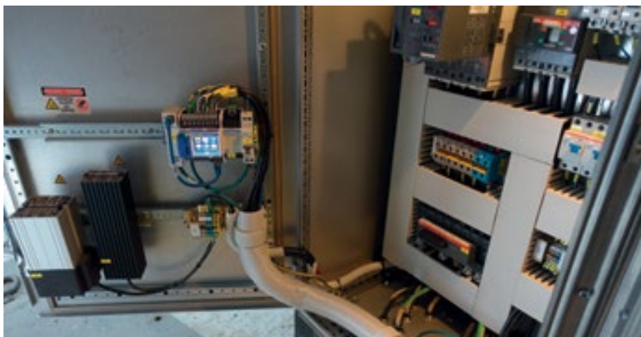
The Power Monitoring System installed in the pedestal of a European ALMA antenna.
