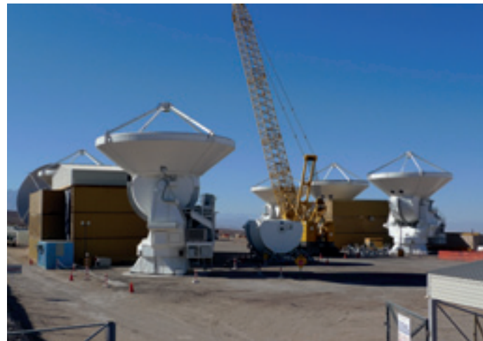
By the end of 2010 six antennas were assembled. Installation of the seventh reflector started in the shelter.
