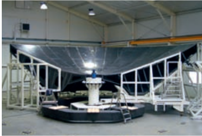
Assembly of the first Backup Structure.
