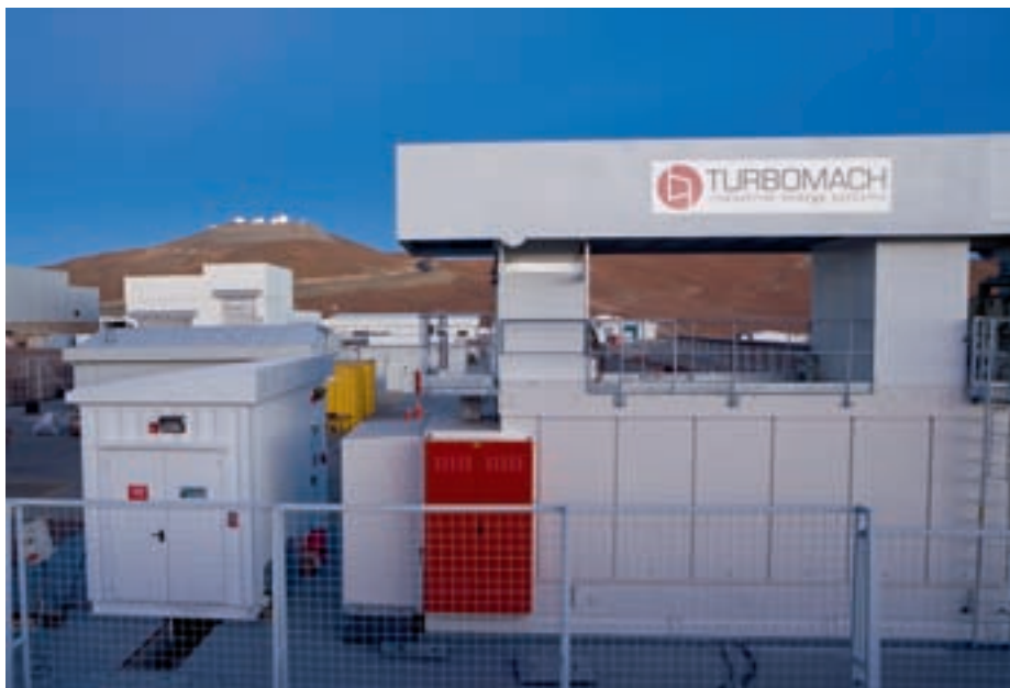
The multi-fuel power station.
