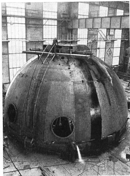
Fig. 9: Dome for 1.5 m Spectrographic Telescope in the Works of Seibert-Sécométal in Saarbrücken. Circular holes for large ventilators visible.
