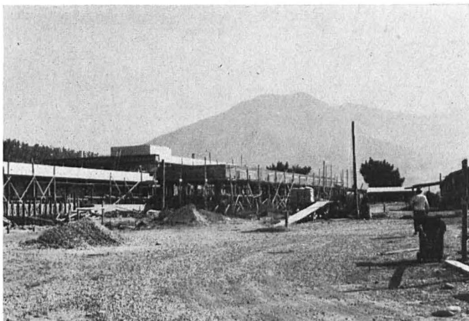
Fig. 16: ESO Headquarters in Santiago: Main Building, northern part of east façade.
