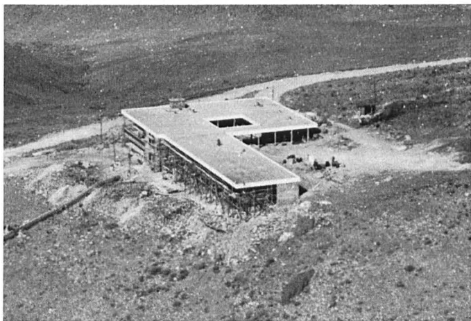
Fig. 4: Hostel on La Silla under construction.
