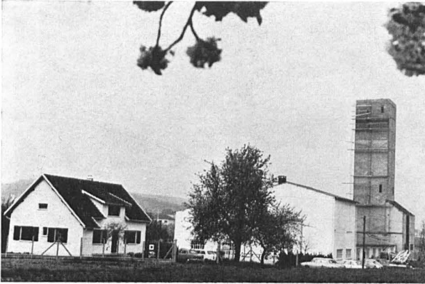
Fig. 20: Works of REOSC at Ballainvilliers near Paris with tower for optical tests under construction.
