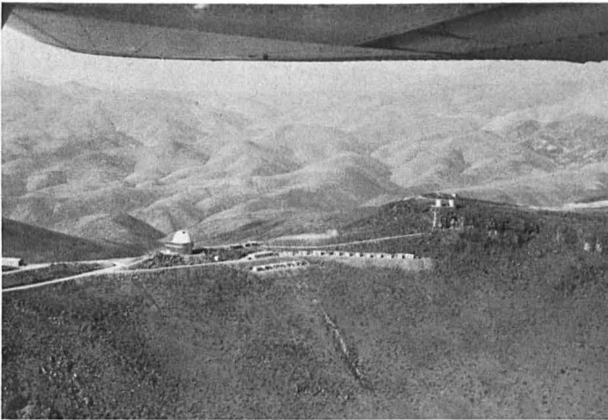
Fig. 2: Air view of La Silla from south-west: Main Summit and Second Summit, right. Schmidt Building and La Silla Camp, near centre. Workshop, left edge.
