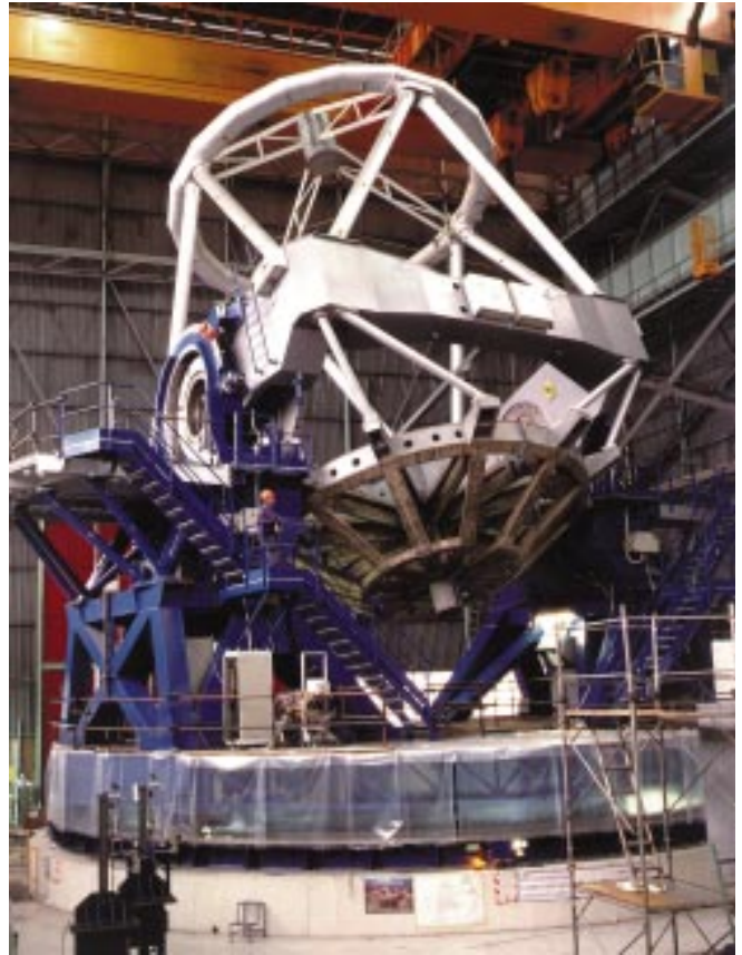
Figure 5 shows a different view of the telescope structure of the first telescope, and clearly visible is the dummy simulating the mass and other characteristics of the mirror cell and associated mirror. This piece in steel and concrete was extensively used to test the procedure of mounting and dismounting the mirror cell.
