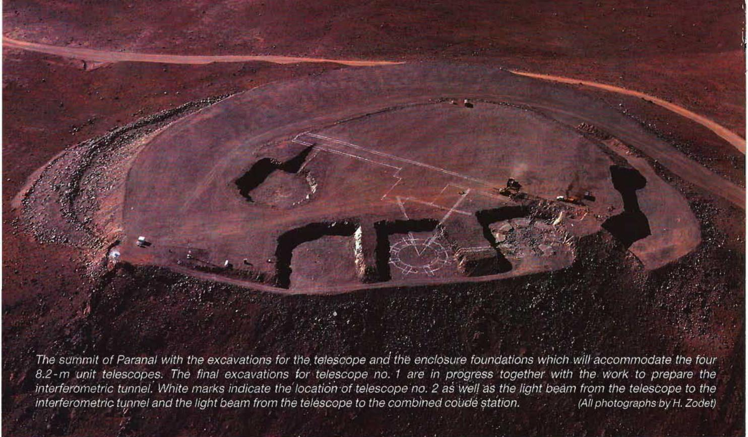
The summit of Paranal with the excavations for the telescope and the enclosure foundations which will accommodate the four 8.2-m unit telescopes. The final excavations for telescope no. 1 are in progress together with the work to prepare the interferometric tunnel. White marks indicate the location of telescope no. 2 as well as the light beam from the telescope to the interferometric tunnel and the light beam from the telescope to the combined coude station. (All photographs by H. Zodet)
