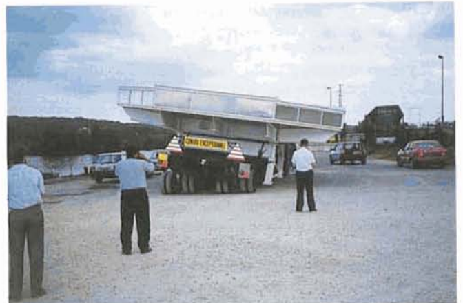
Figure 3: "Rock-and-roll" test on the hydraulic platform.
