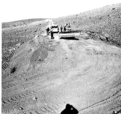
June 1965: Road construction on La Silla.
