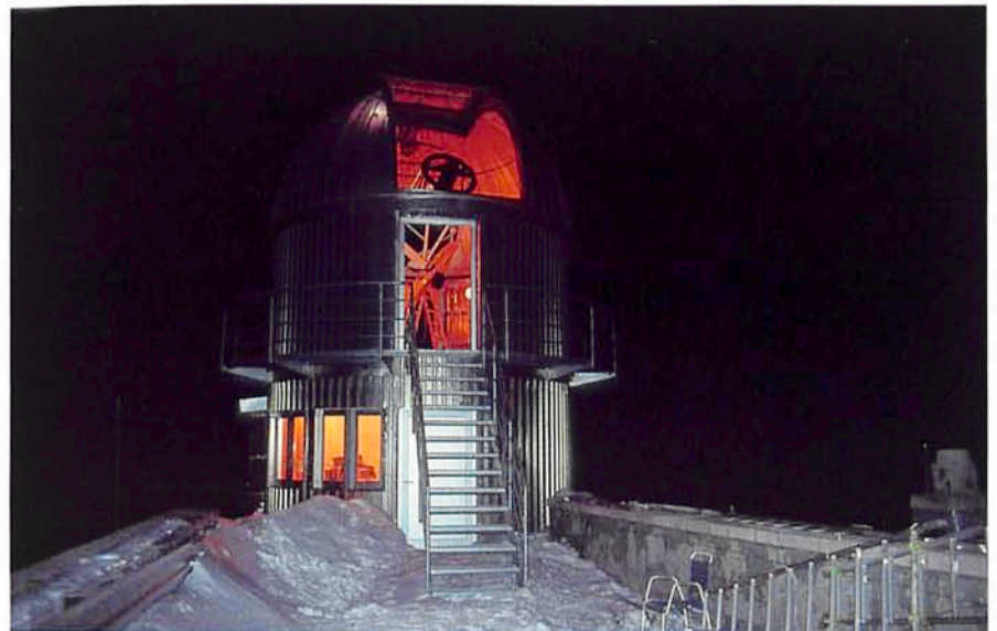
Figure 1: Ready for observation: the new telescope on Mount Wendelstein.
