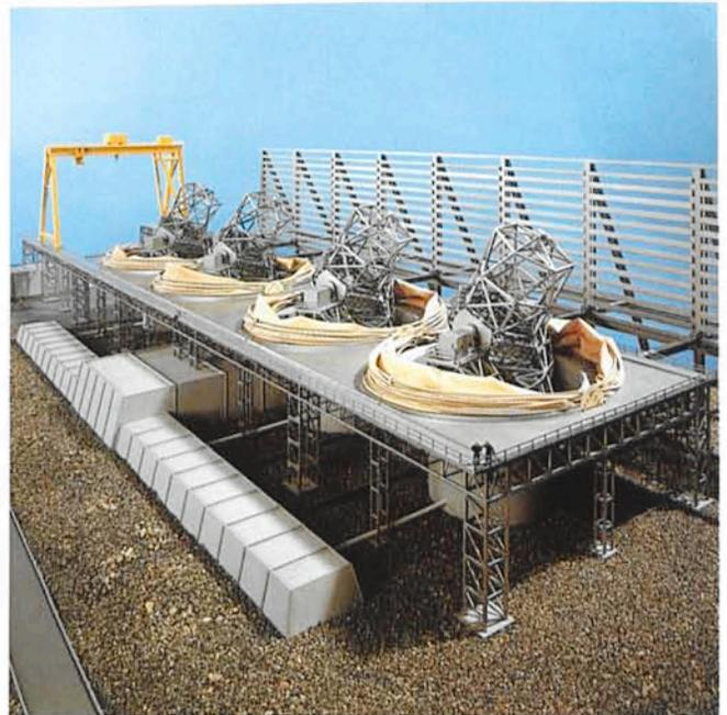
Figure 2: *Second iteration: inflatable domes, a lighter platform.*
