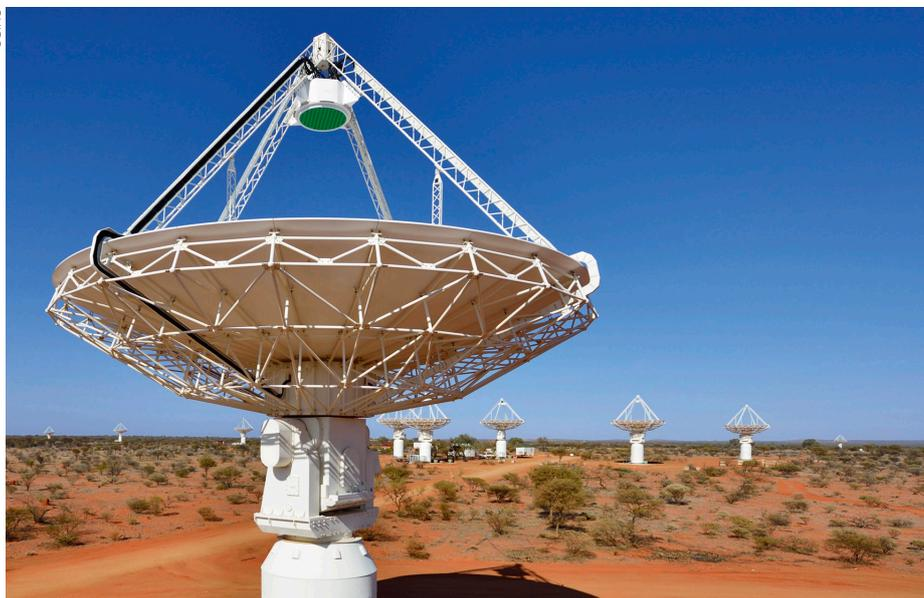
Figure 4. 12-metre antennae of the Australian Square Kilometre Array Pathfinder in Western Australia.
