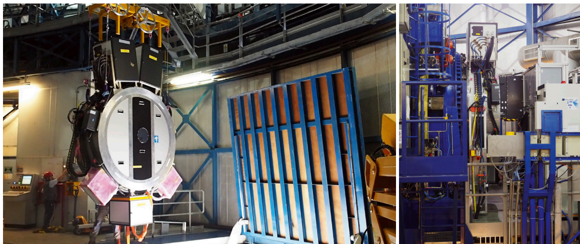
Figure 7. Left: GALACSI being hoisted through the azimuth hatch after transport from the Paranal New Integration Hall to UT4. Right: The very tight margin to manoeuvre this sensitive module between the Nasmyth acquisition and image rotator unit and the MUSE fore-optics can be seen.
