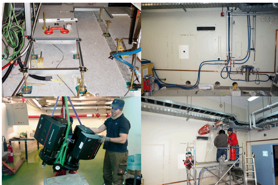
Figure 4. An album of work in progress for the VLT upgrade: installation of the new false floor covering the cable trays running from the instruments (upper left); installation of a new cooling distribution system in the Combined Coudé Laboratory (upper right); integration of a more powerful pump to provide cooling for the second generation instruments (lower left); drilling of a new feedthrough between the Combined Coudé and the VLT Laboratories (lower right).
