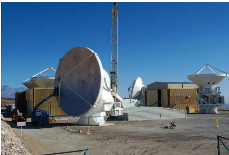
Figure 3. The AEM antenna camp at the OSF. Five antennas are fully assembled while a sixth is inside the temporary shelter on the right ready for the installation of the main reflector assembly; parts of the seventh antenna are also being assembled.
