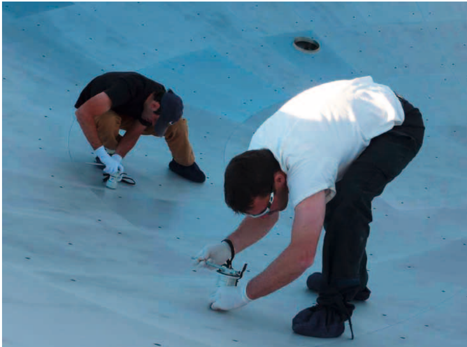
Figure 5. Adjusting panels on the AEM antennas using the manual panel adjuster tools. Note that this operation can be performed walking on the reflector surface when the antenna is stowed; the hole on the dish surface to the rear of the image is used for the optical pointing telescope.
