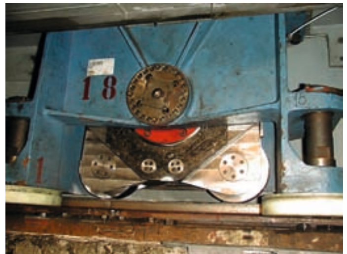
Figure 7: One of the eight new wheel units is shown in position attached to the dome.
