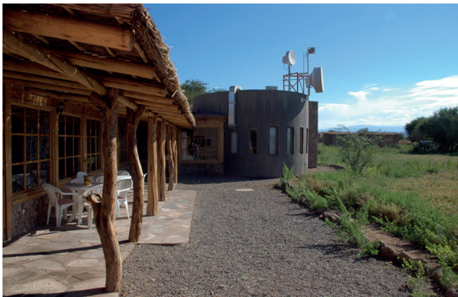
Figure 3: The APEX control room in the Sequitor base, from which Claudio Agurto operates the telescope (lower left). The radio link transmitters are visible on top of the building. To the left, the laboratory wing is seen, with our open air meeting room.
