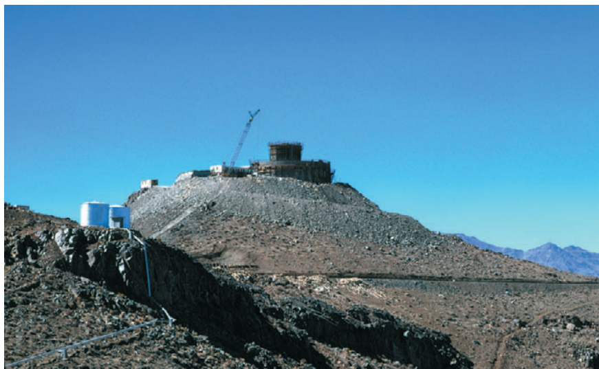
Construction of the building for the 3.6-m telescope at La Silla in 1975.
