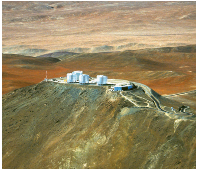
... and after construction of the VLT .
