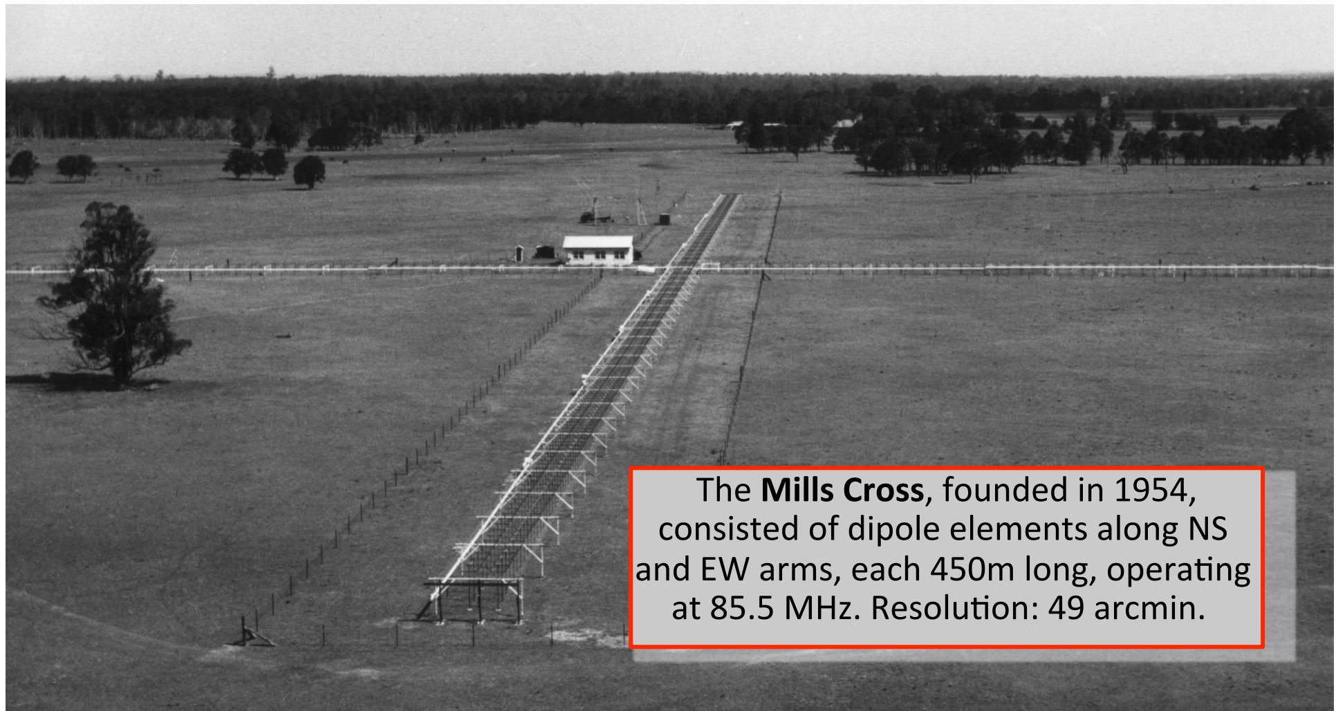
The **Mills Cross**, founded in 1954, consisted of dipole elements along NS and EW arms, each 450m long, operating at 85.5 MHz. Resolution: 49 arcmin.
