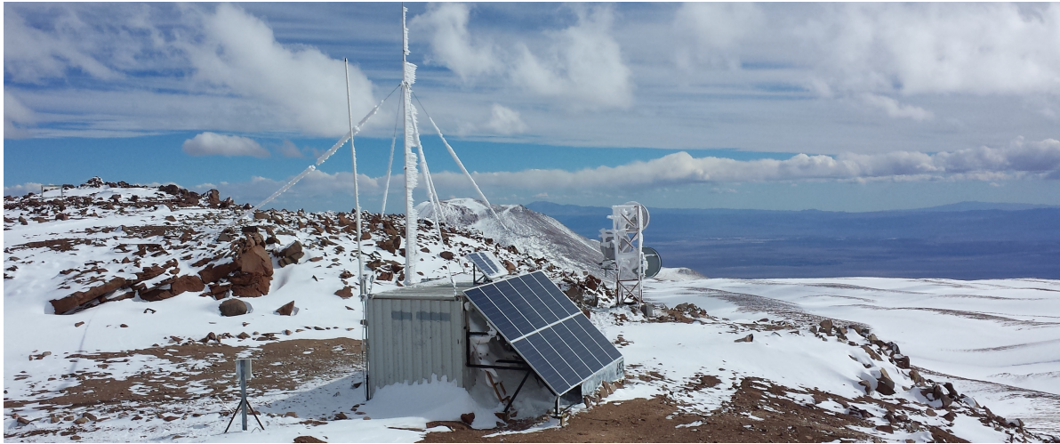
Figure 6: At the summit of Cerro Chico, 1.5km away from the telescope, the radio link antennas are directed to the APEX basecamp with a direct 45.5km line of sight. The photo shows the MWL antennas on the right side in the background. In the foreground the panels of the solar plant are visible, mounted on the lee side of the container. Therein, a small thermally isolated compartment is built that hosts the electronic equipment of the link and the solar plant. The equipment's heat dissipation keeps the temperature of the battery bench above -10^{\circ}\text{C} at outside wind-chill temperatures of -40^{\circ}\text{C} . Not visible on the photo is the 25dB gain Yagi antenna of the backup LBL, mounted on the same pole as the MWL antennas.
