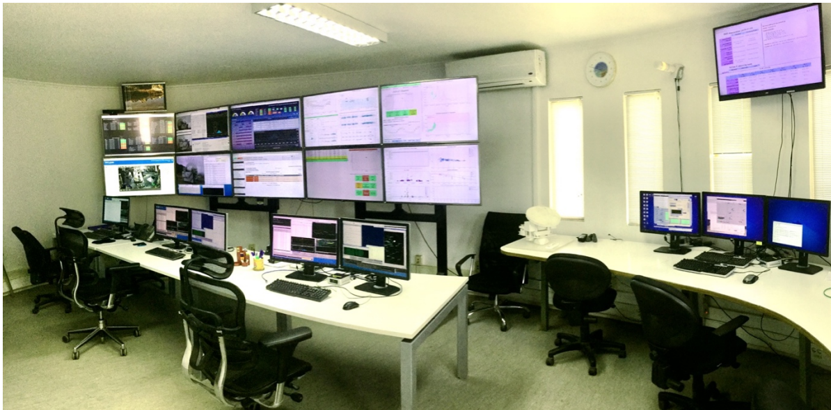
Figure 10: Sequitor control room for Sciops-R operations. On the left area, the observing team has available the observing tools and monitoring information to conduct science operations. The engineer on duty has assigned a working station where he can monitor the systems and coordinate actions with the observing team and the high site engineer. The right area is used by visiting observers who can work while following up the course of the observations.
