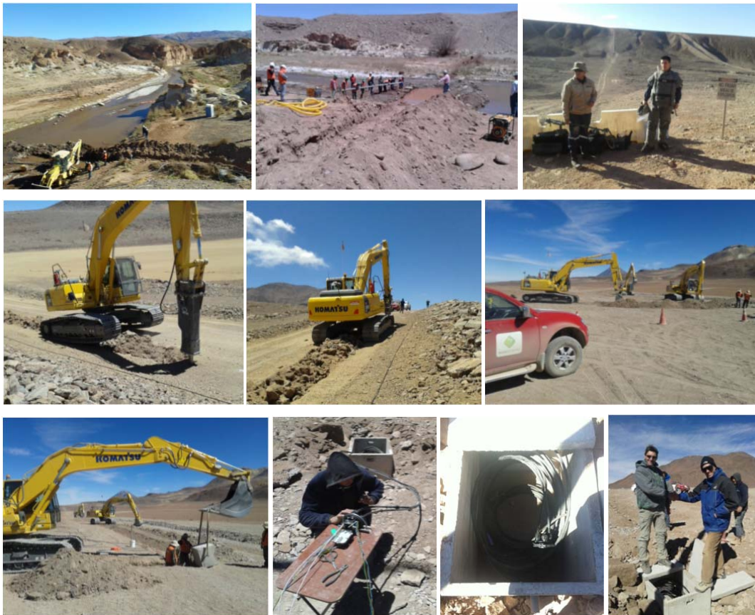
Figure 4: Various moments of the construction of the fiber cable. From the top left, crossing of the San Pedro and Vilama rivers; specialists from the Chilean Army clearing one of the minefields; opening the trench for the cable and installing the chamber for the splice box; final splicing of the ALMA fiber pair into the connection to the Observatory; final handshaking between the SILICA and ALMA Project Managers.
