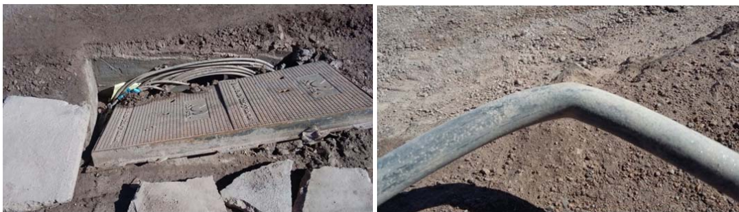
Figure 15 damaged chamber and fiber cable in Calama
