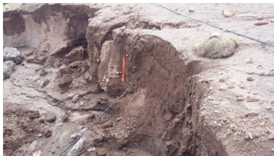
Figure 13 fiber cable section exposed by the rain.
