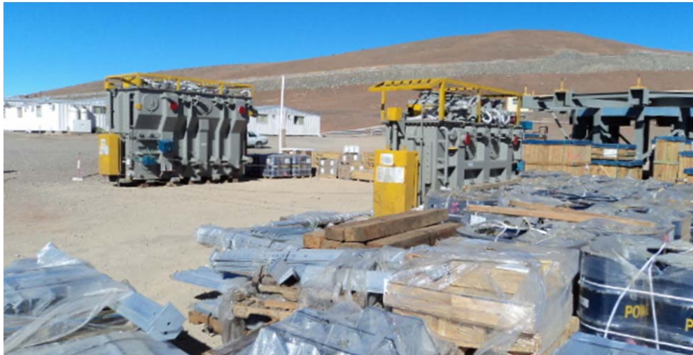
Figure 7: The 220/66kV and 66/23kV transformers and other material for the grid connection.
