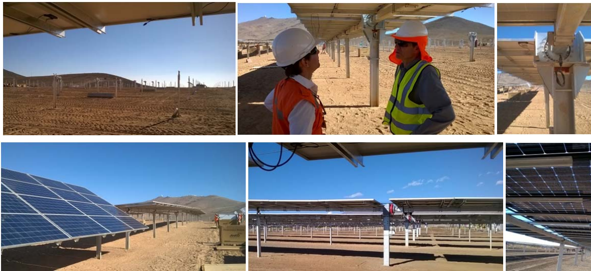
Figure 3: The structure sustaining the panel with the rotating table and a detail of the bifacial modules..
