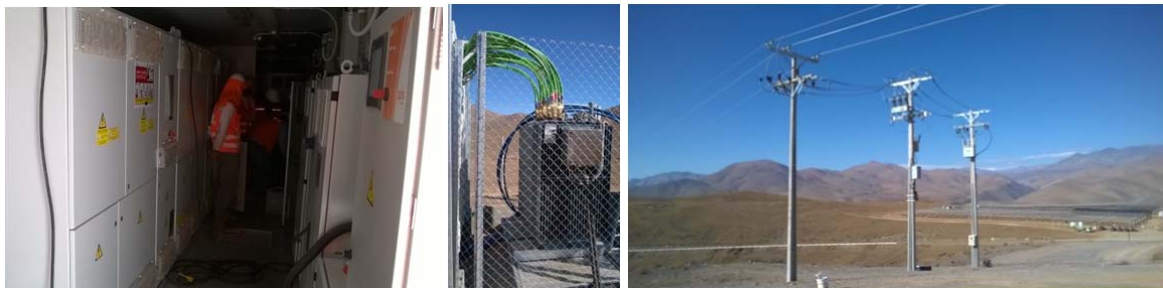
Figure 4: Inverters, transformer, and connection to 23kV medium voltage line.
