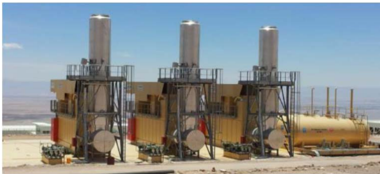
Figure 8: The ALMA power generation system consisting of three multi-fuel turbines.
