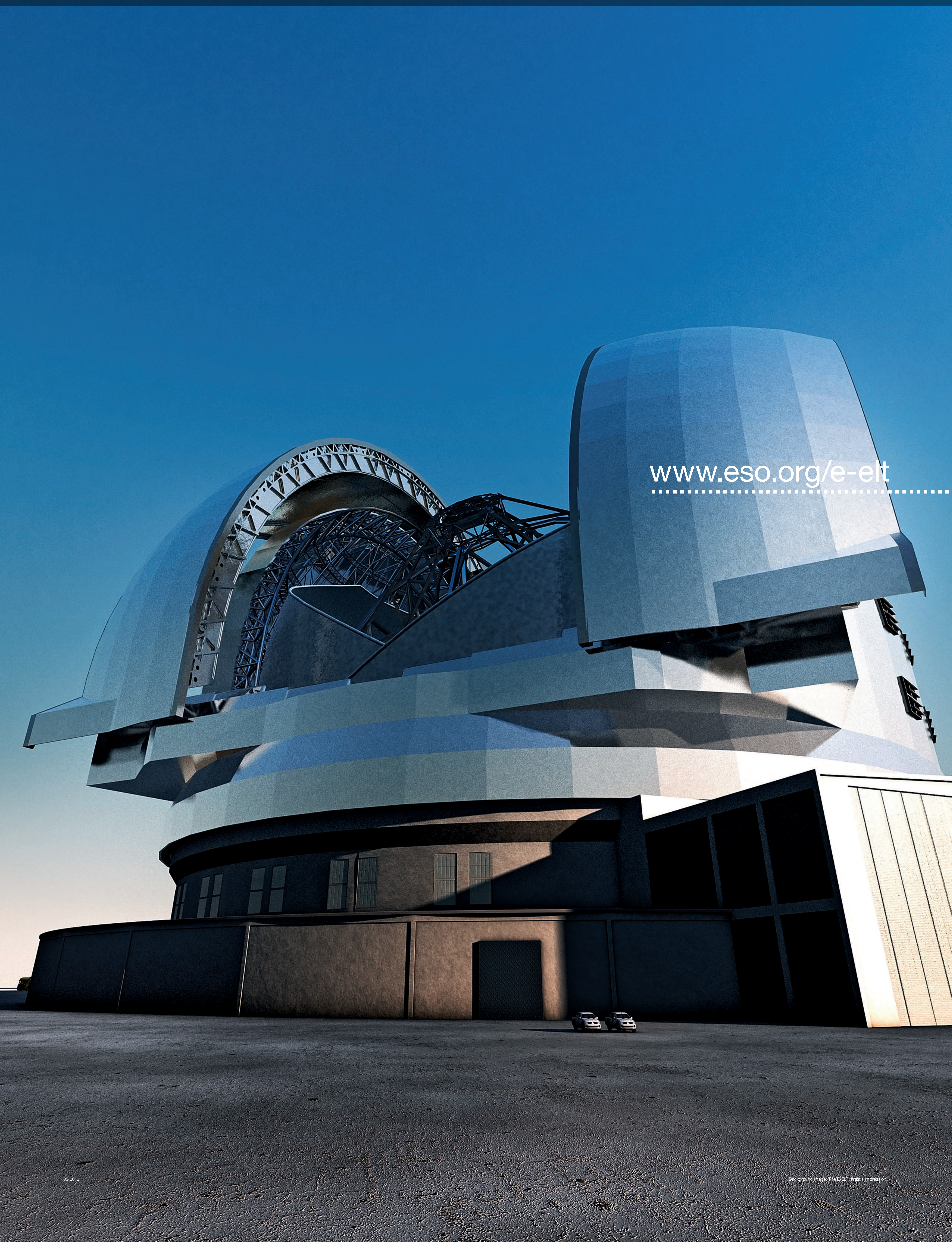
The 40-metre-class E-ELT, with its huge segmented primary mirror, is based on a revolutionary five-mirror concept.
